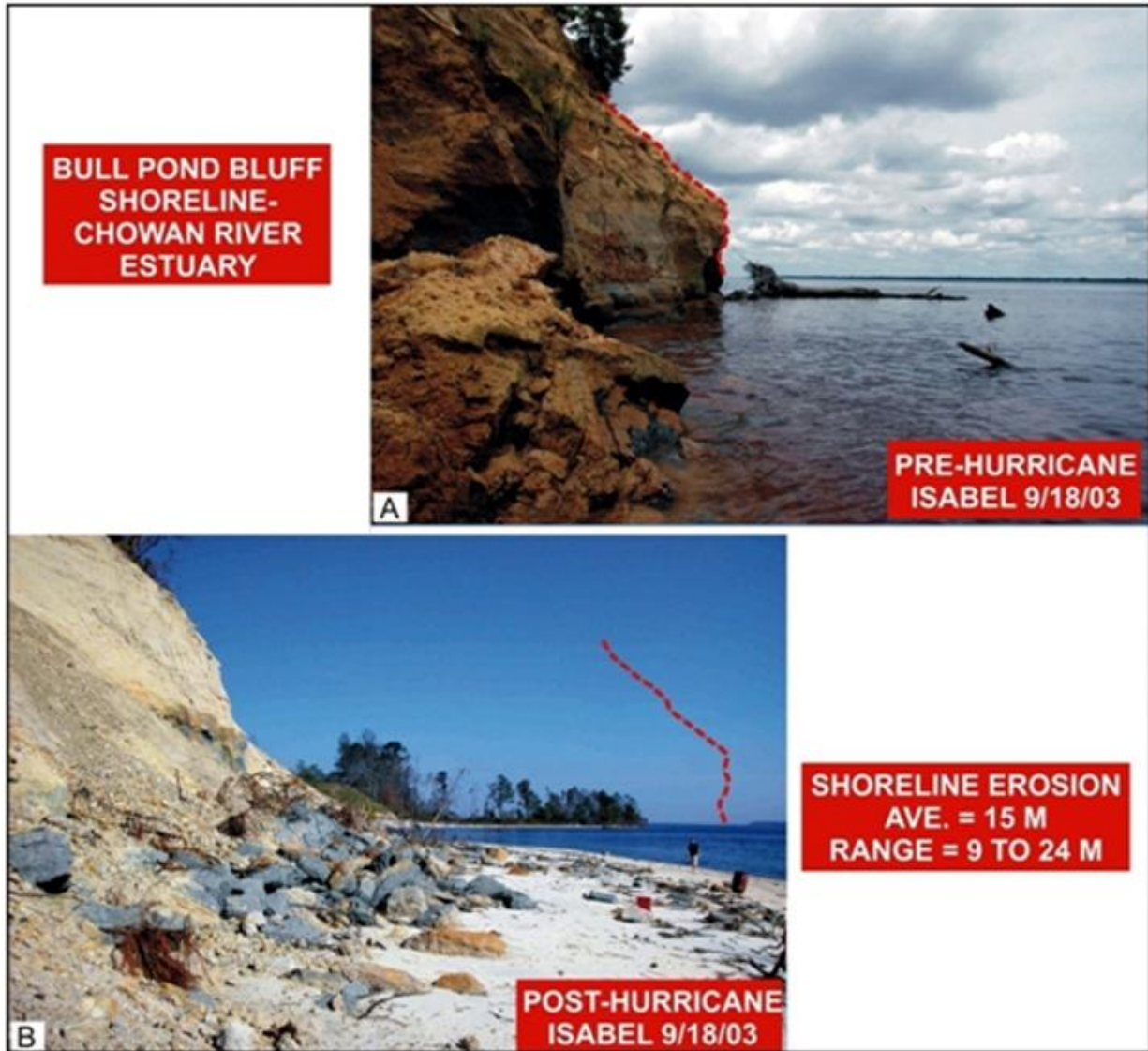
Figure 1-30. Two photographs of an eroding estuarine sediment-bank shoreline along the western side of the Chowan River. Panel A: Pre-Hurricane Isabel photograph was taken prior to the storm on September 18, 2003. This ~75-foot high bluff consists of a lower clay bed (~30 feet thick) with an overlying sand bed (~45-50 feet thick). Panel B: The post-Hurricane Isabel photograph was taken on October 6, 2003 from about the same location along the bluff shoreline as Panel A. The red dashed line in Panel A is in the same relative location as in Panel B. The average bluff shoreline recession was about 50 feet (range from about -30 to -80 feet) for the several segments of accessible bluff shoreline. Figures are the front and back cover of Riggs and Ames (2003).
